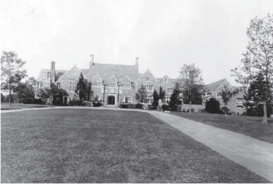
FIGURE 6: Thomas S. Dignan residence, The Great Road, 1930–1931. Bauhan Collection.
